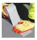
Peel the release liner and apply the tape to the prepared surface
