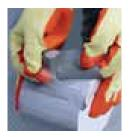
Push fingers back together allowing the release liner to come away from the tape backing
